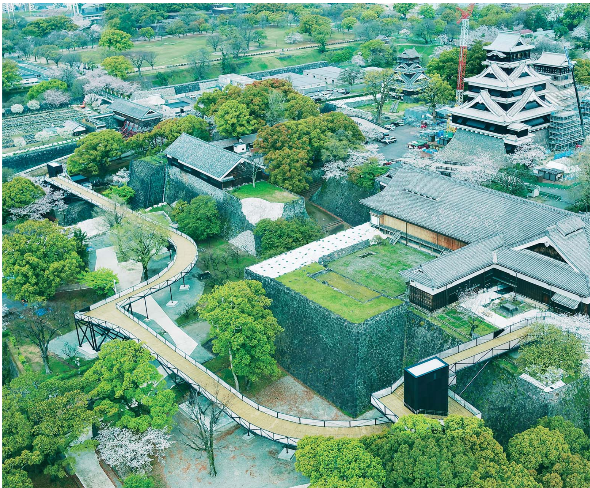
復旧工事そのものを見せる、全長350mの熊本城特別見学通路を見る空撮。写真右に熊本城天守閣と本丸御殿大広間。 Drone view of the 350m long Kumamoto Castle Reconstruction Observation Path for the viewing of ongoing restoration works. Kumamoto Castle Tenshukaku (Main Keep Tower), Honmaru Pavilion Grand Hall on the right.
