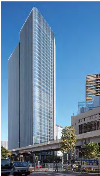
設備バルコニーで意匠的に分節した首都高速側のファサード Façade on Metro Expressway Side Articulated by Mechanical Equipment Balconies
