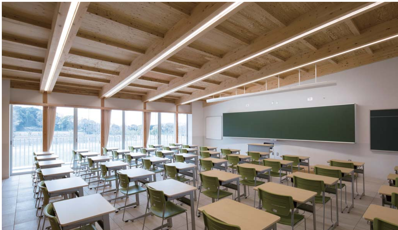
木造ゲルバー梁架構の2階普通教室 | 2nd Floor Classroom with Wood Gerber Beams Spans
