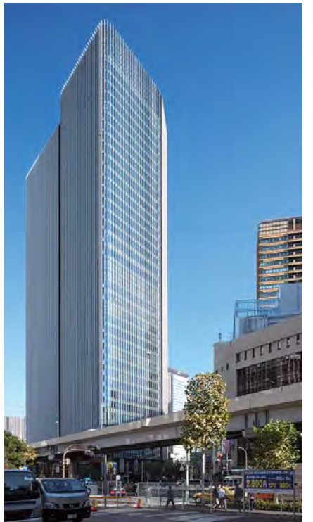
設備バルコニーで意匠的に分節した首都高速側のファサード Façade on Metro Expressway Side Articulated by Mechanical Equipment Balconies
