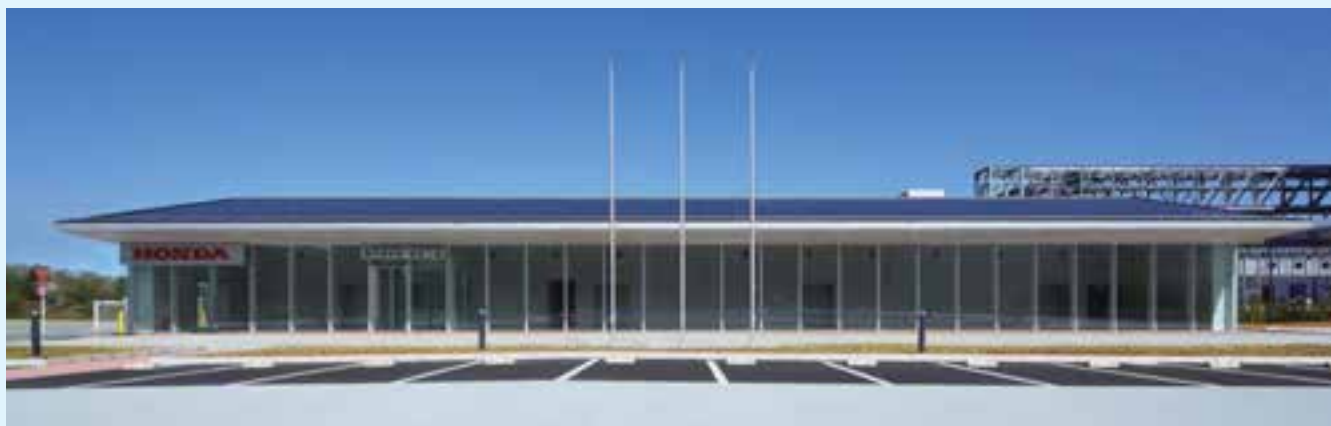
太陽光パネルと一体的に収めた大屋根による熱負荷の抑制 | Reduction of Energy Loads through Use of Solar Panels Integrated into Grand Roof
